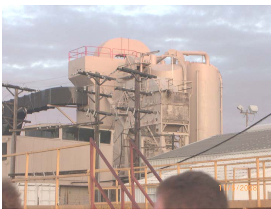
This is the control center to the barrel furnace.
