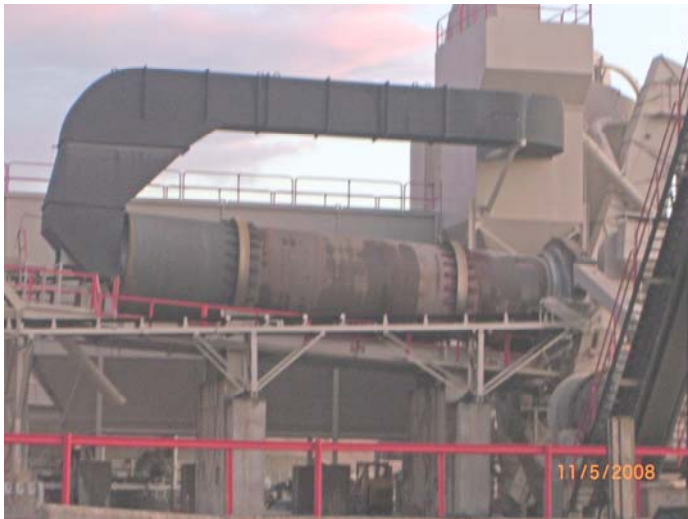
The barrel furnace melts the asphalt
